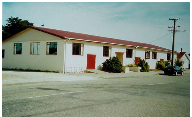
The building purchased by GPC Gore
