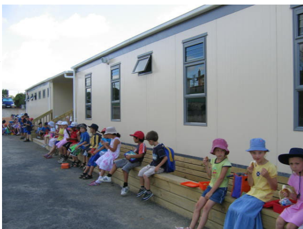
Manukau Christian School—buildings now complete
