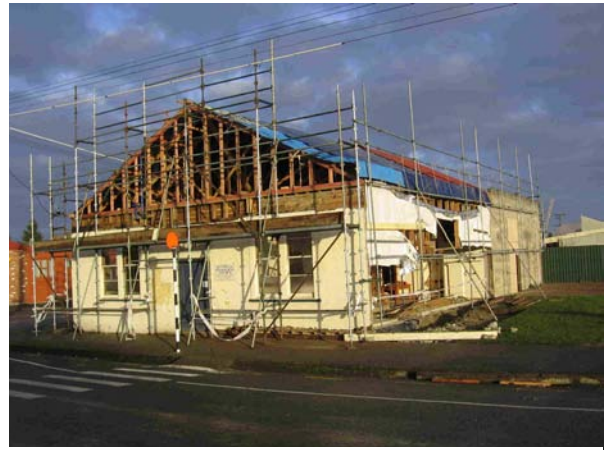
Wyndham Evangelical Church's building renovations
