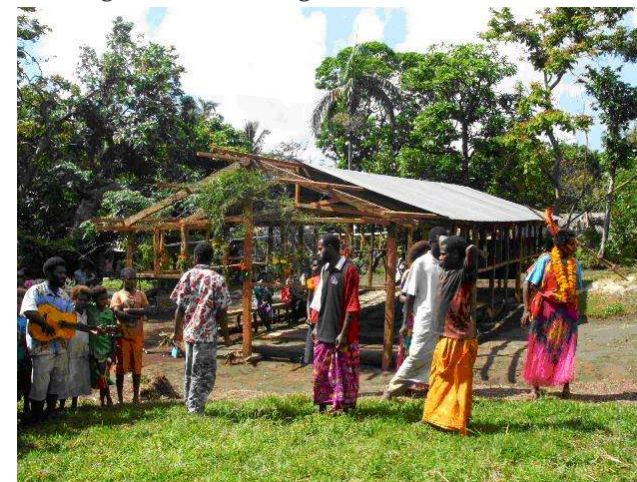
Chapel under construction in Vanuatu
